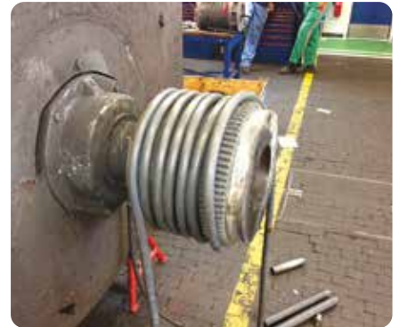
Heating a coupling for dismounting
